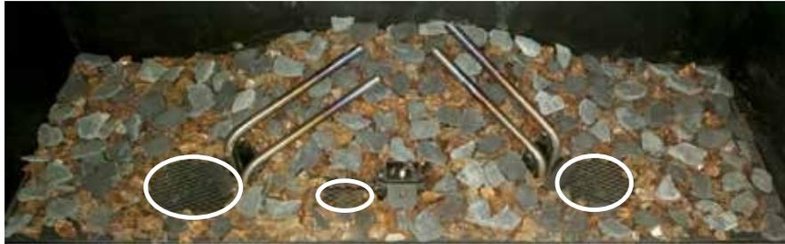
1. Arrange fire glass in the above configuration. Ensure that glass is not placed in circled areas.
