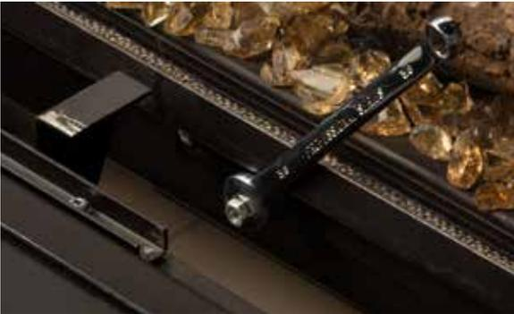
1. Loosen the coupling nuts on the bottom front glass bracket using a small wrench or socket set. Do not completely remove.
